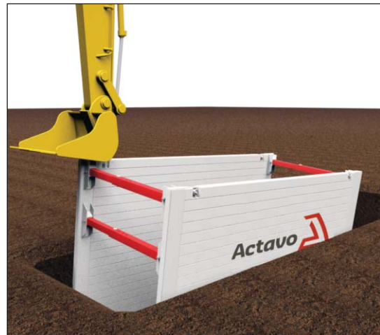
Stage 4: Push each corner in turn until the box reaches the limit.
