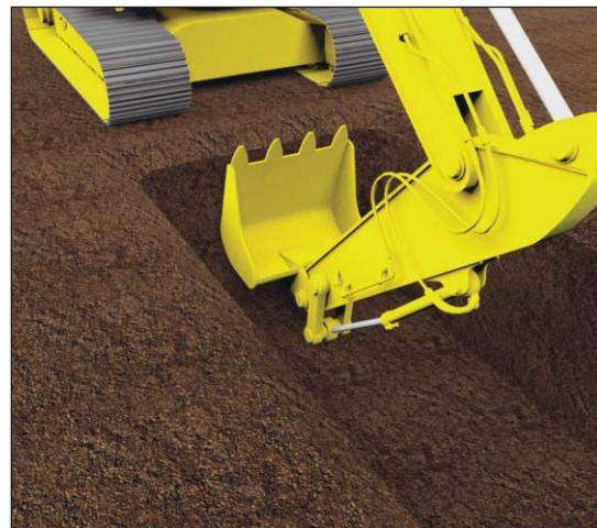
Stage 4: Dig in front of the box.
