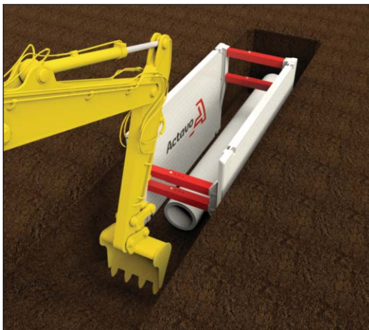
Stage 3: Lay the first pipe.
