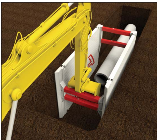
Stage 3: Lay the first pipe.
