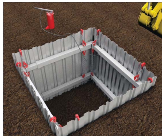
Stage 6: Pump braces with Shoring fluid to hold in place. Once complete, install Ladder Access and Guardrails. Enter excavation once safety is declared.
