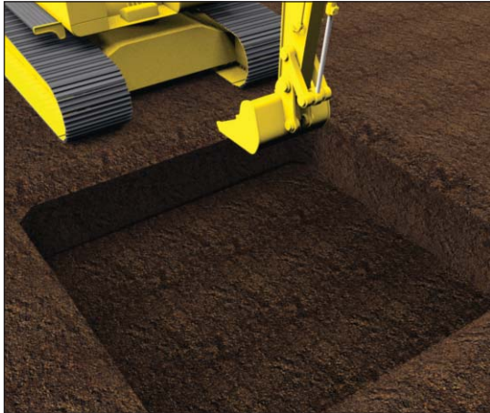
Stage 1: Dig a Shallow Excavation.
