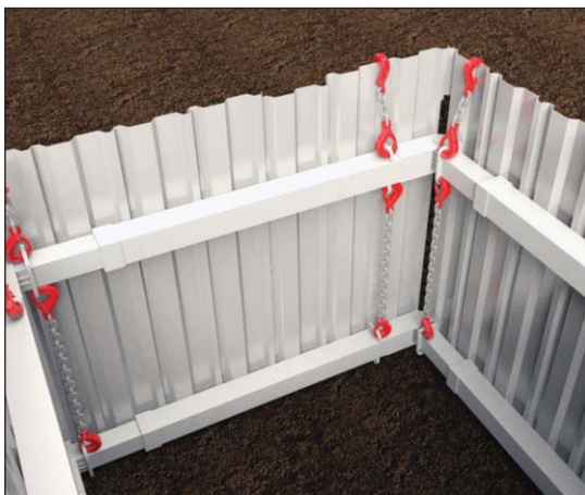
Stage 5: Attach holding chains to each brace.
