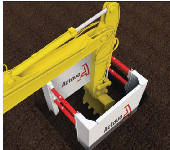
Stage 4: Excavate beneath the panel and remove any excess material.
