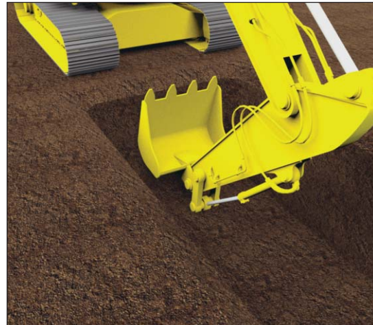
Stage 4: Dig in front of the box.
