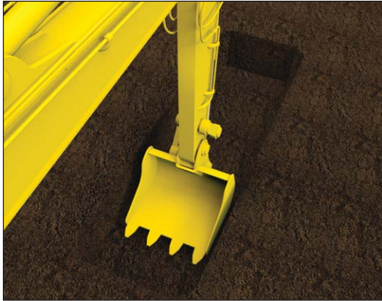
Stage 1: Dig the starter trench.
