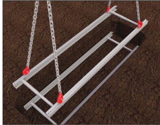
Stage 2: Lower the frames into the trench on top of each other.
