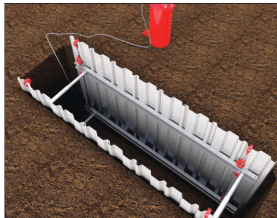
Stage 6: Pump the frames to prevent trench instability.
