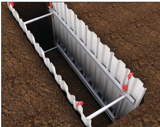
Stage 5: Dig below lowest frame, drive in the remaining trench sheets and add restraining chains.
